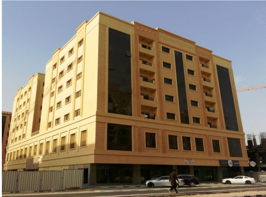
Project : PROPOSED (G+2P+5) RESIDENTIAL BUILDING PLOT NO 5091 (7/695), MUWAILAH, SHARJAH Client: AL WALEED KHALID BIN KHADIM Consultant: AL NAHDA ENGINEERING CONSULTANT
